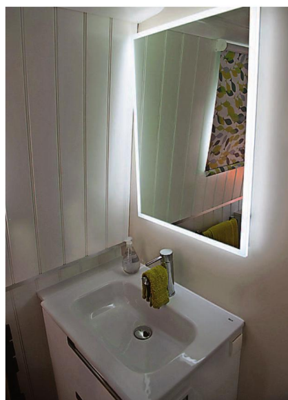
The vanity unit is fitted with a basin by Roca
